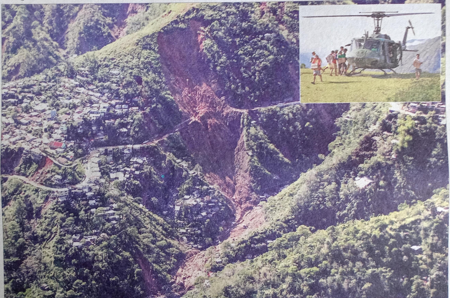
THE WRATH OF TYPHOON OMPONG – A huge landslide that hit a mining village in Ucab, Itogon, Benguet at the height of Typhoon Ompong left 59 dead and 42 others missing as of Sept. 21, 6 p.m. Authorities reported that the death toll in the Cordillera due to landslides has reached 83 while 45 others are missing. With many villages still isolated due to landslides, the Philippine Air Force has been conducting aerial relief operations in Benguet while public and private donors are reaching out to those affected by the super typhoon (More images of the Typhoon Ompong aftermath on pages 14 and 15). -- Harley Palangchao
